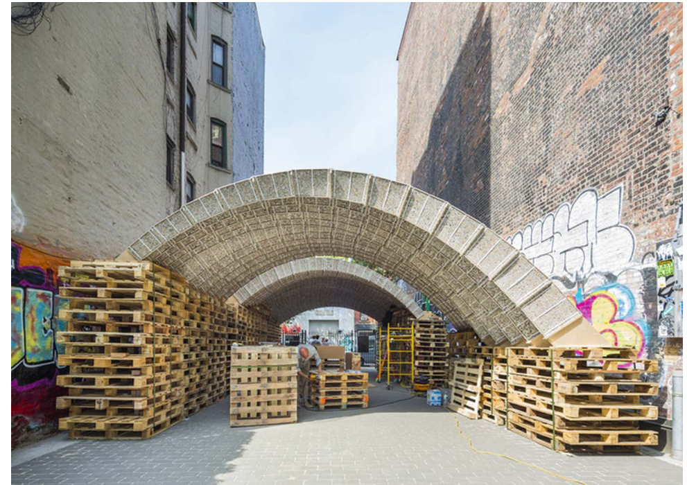
Fig. 8: Hebel's EHT pavilion, made from used drink cartons
