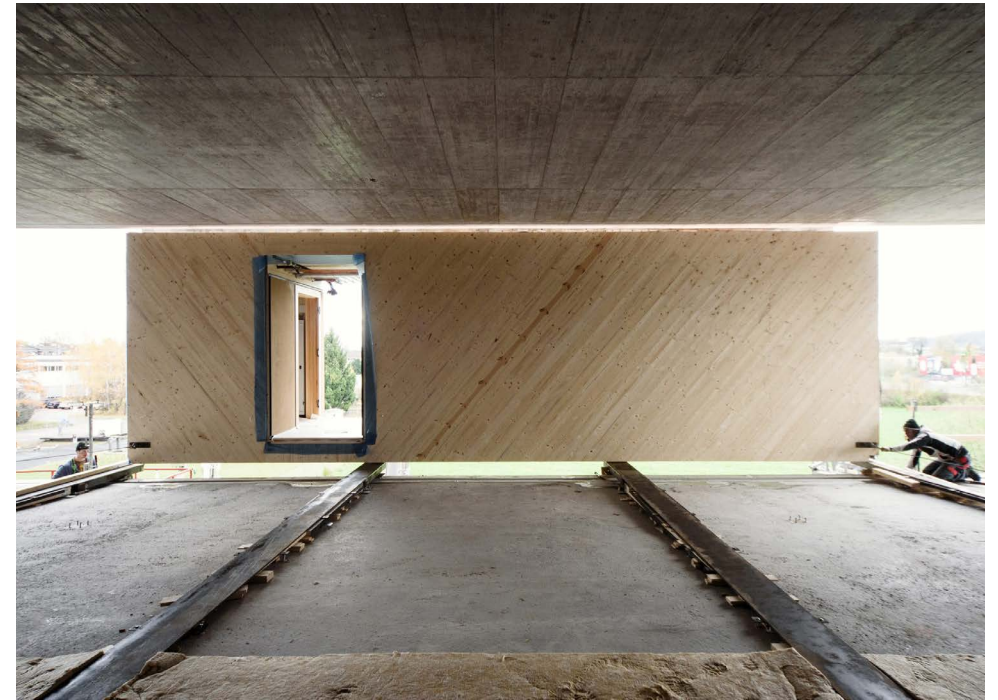
Fig. 11: photograph showing the construction process, with elements positioned by cranes and rails
